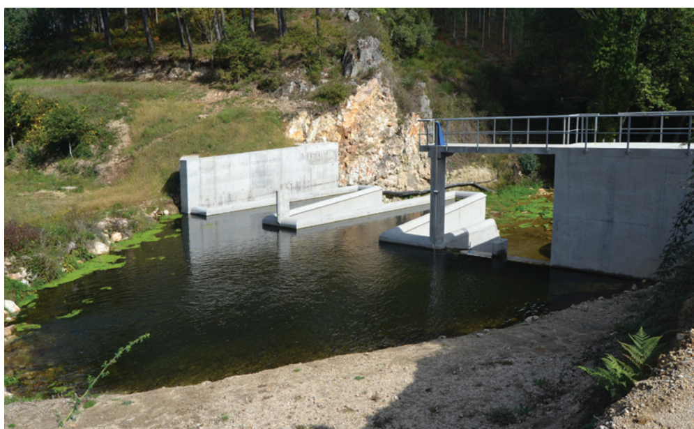
Weir and labyrinth spillway chute. Upstream view
