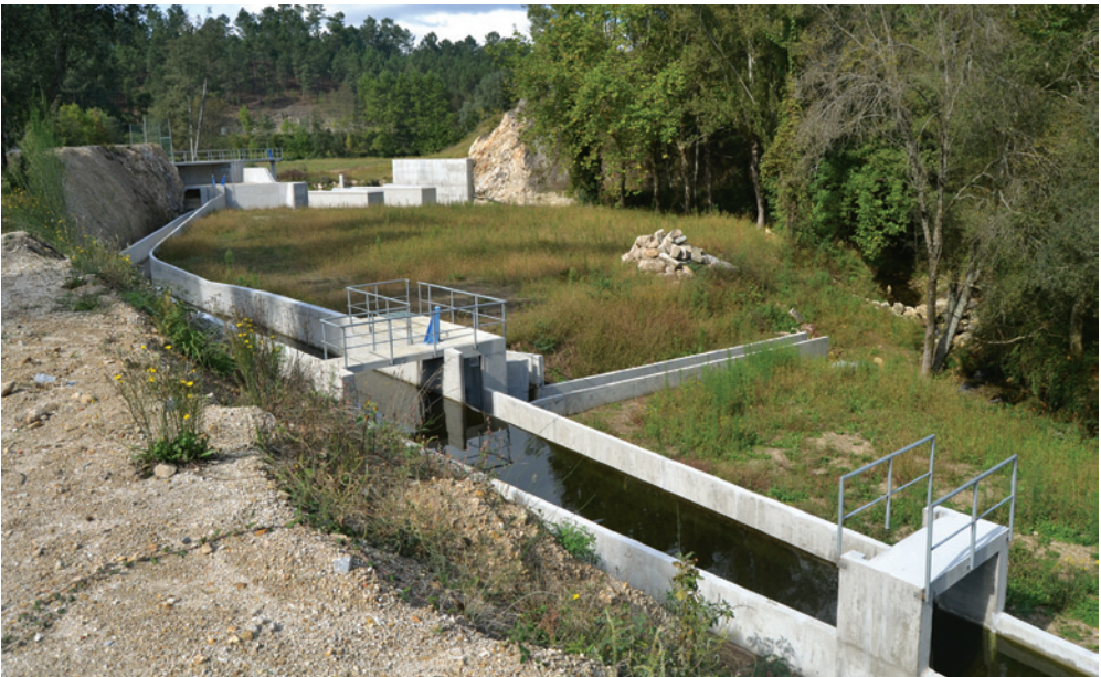
Weir, desilting plant, lateral spillway and water intakes for irrigation
