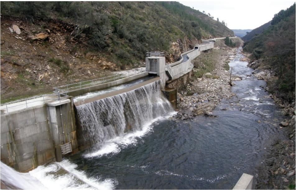
Hydraulic circuit downstream of the weir on the Tinhela River. From upstream to downstream: sluice gate of the pebble-removing system, lateral spillway and maintenance discharge, operating mechanism of the flat gate designed to isolate the diversion canal and initial reach of such canal
