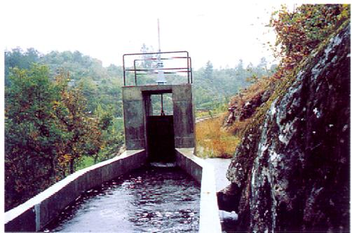
The hydraulic circuit extends along Covas river's right bank and Couto river's left bank. In its free surface branch, between the weirs and the forebay, it is composed of two reinforced concrete canals, with a global length of 3 200 m, and 0,85 m and 2,80 m wide rectangular sections.
