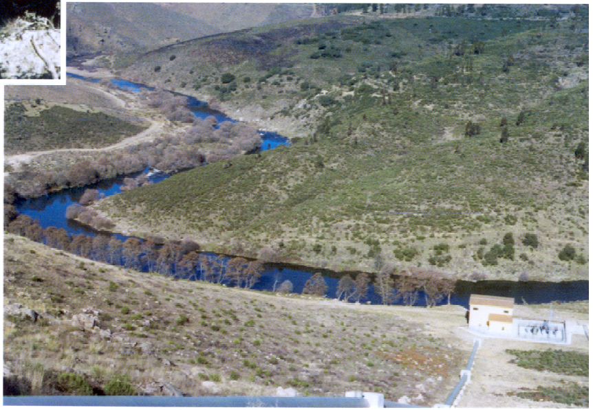
Penstock and powerhouse
