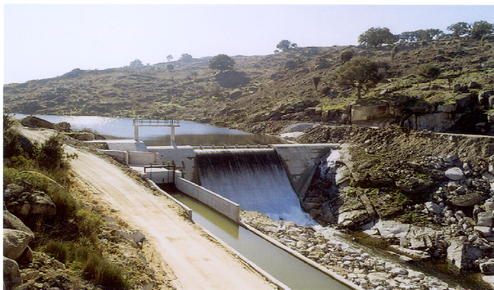
Cabras weir and initial stretch of the Cabras-forebay canal
